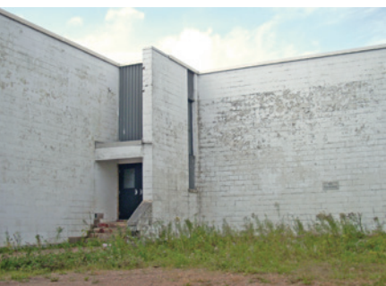
Photo 4 – The old Oxford school prior to development.
