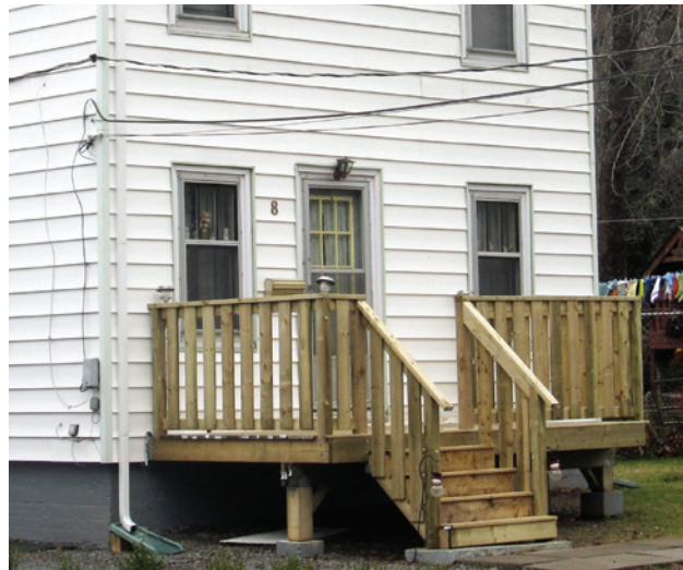
Photo 2 – Home with new porch, gutters, and siding.
