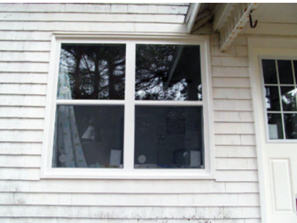
Photo 1 – Home with new window and exterior door.
