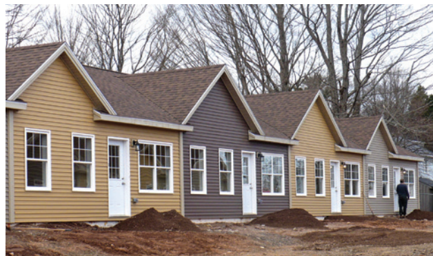
Photo 3 – Our investments enabled a private developer, in Truro, to build a 14-unit one storey rental townhouse project.
